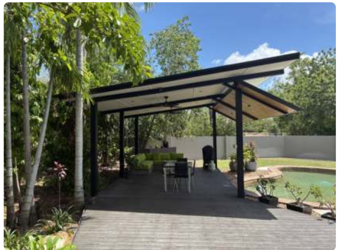
590-4080-7 Gazebo, Decking & Blockwork fence
