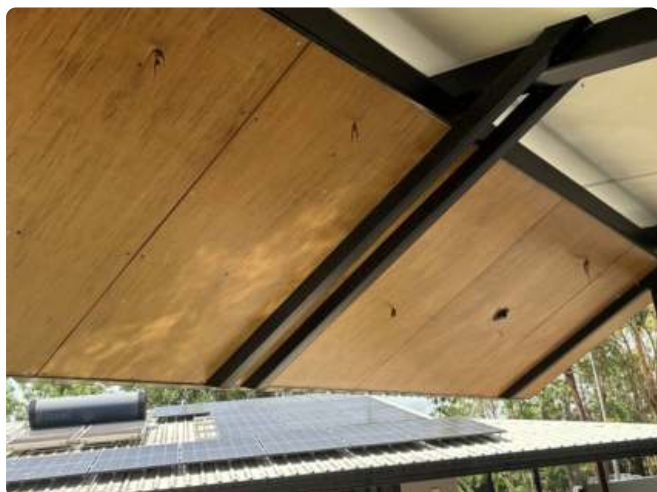
Decking boarder is bowing and peeling away from subframe.
