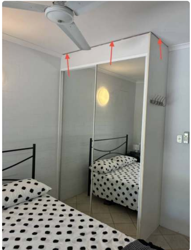
Noticeable gaps between wardrobe and ceiling.
