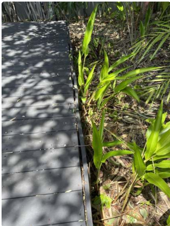
Decking boarder is bowing and peeling away from subframe.
